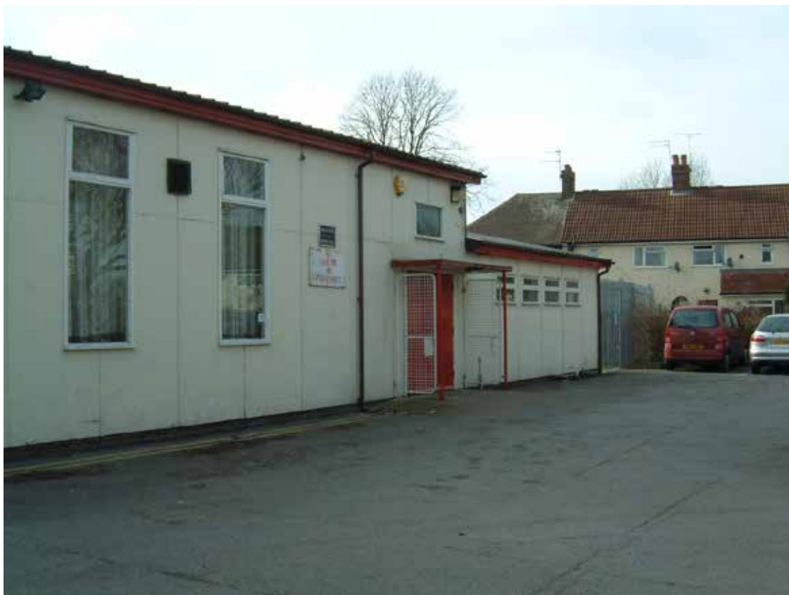
North Hull 'Community Centre, 37th Avenue, North Hull Estate
