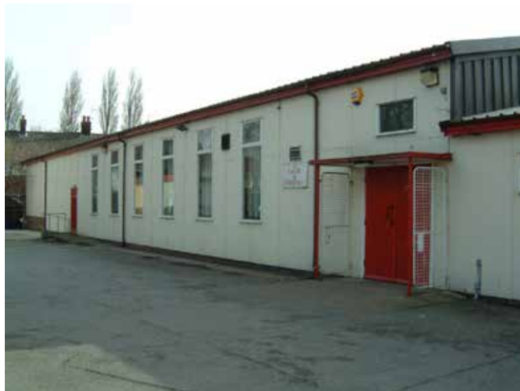
North Hull Community Centre, 37th Avenue, HU6 8AU
